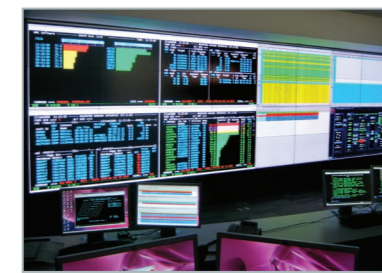
NETWORK CONTROL CENTER Mexico 8 x 4
